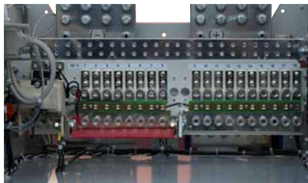
CXPS 48-1T Internal Distribution (053-392-20 with LVD)
